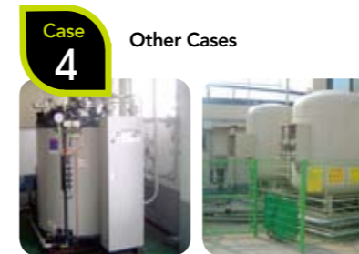
Replacement of boiler fuel
