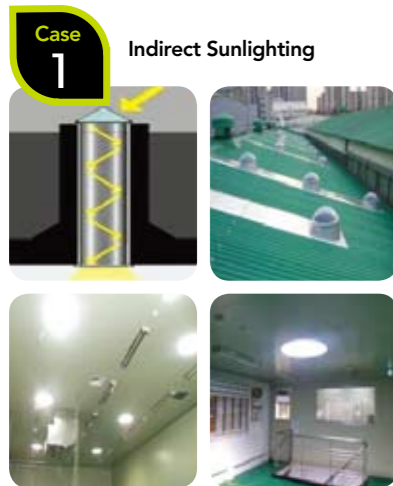
Installation of indirect sunlighting system
