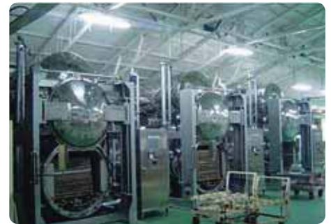
| Installation of hot water-type sterilizer - After |
