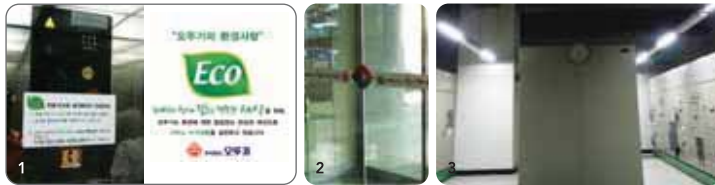
1 Elevator 2 Automatic doors at R&D Center 3 LED lights
