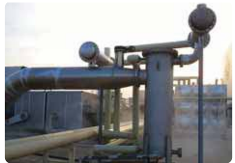
| Waste heat exchanger |
