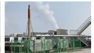
Installation of waste heat recovery system using re-evaporated steam
